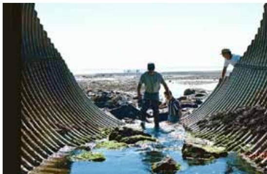
*This aluminum structural plate pipe has handled tidal ocean waters under U.S. Highway 1 at the Bay of Fundy in Maine since 1966.*
