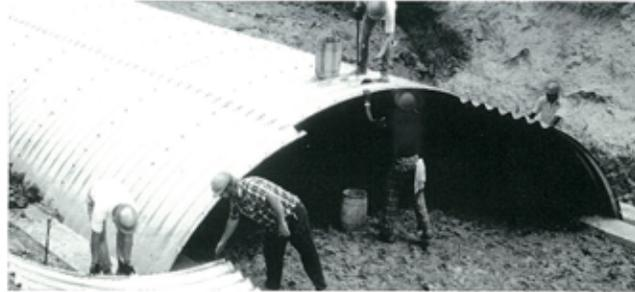
*This 3-plate arch structure assembles nicely into the slotted concrete footing.*
