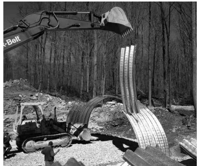
BridgeCor Plate Assembly
