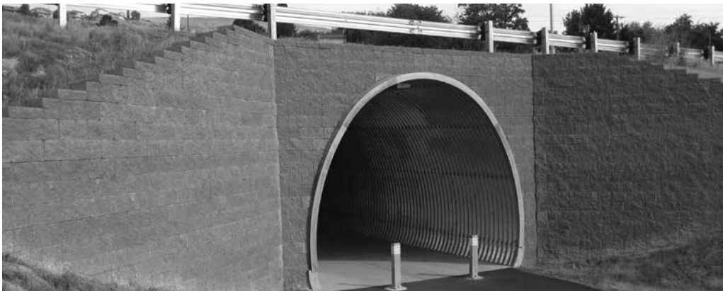
MULTI-PLATE pedestrian underpass with Keystone end treatment.
