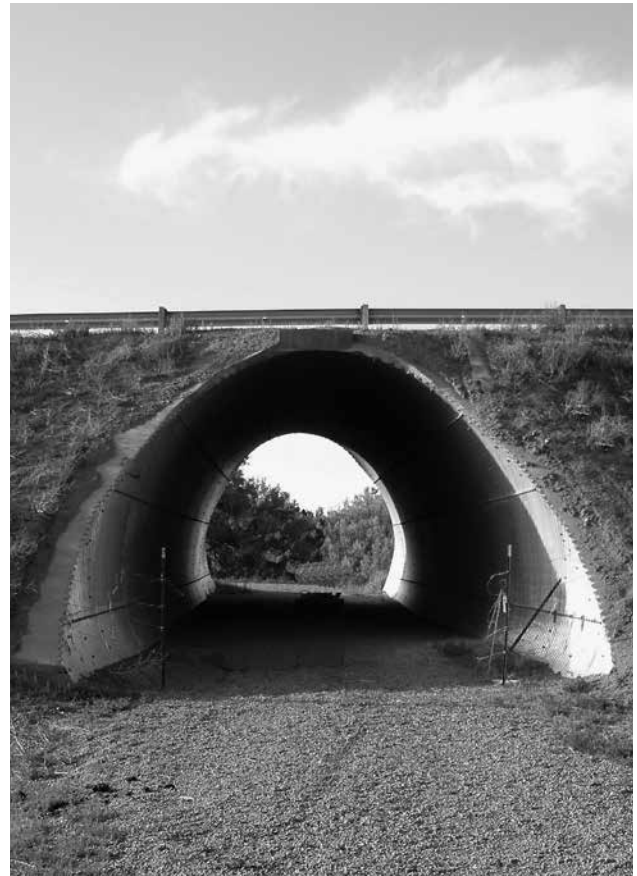
MULTI-PLATE pipe arch is ideal for pedestrian underpasses
