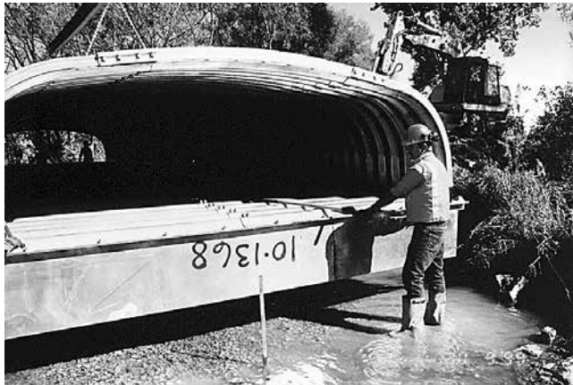
Installation of Aluminum Box Culvert Toewall
