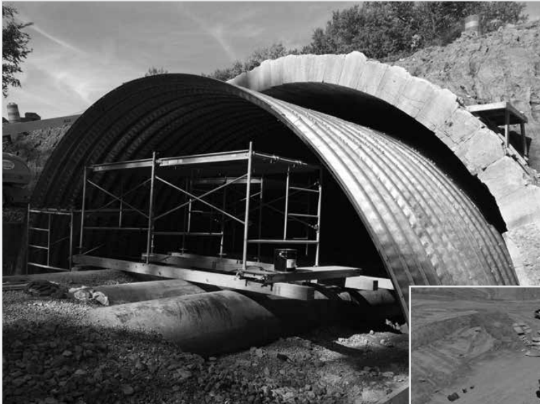
Reline Old Stone Arch Bridges with BridgeCor
