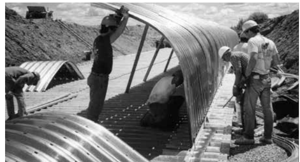
Assembly of ALBC Shell onto Full Invert
