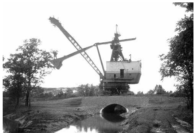
"The Chief" a 5,000,000 lb. drag line over steel SUPER-SPAN™ at Peabody Coal in Zanesville, Ohio
