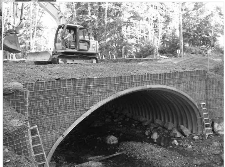
BridgeCor Stream Crossing
