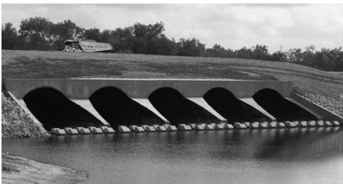
Grade Separation Structure
