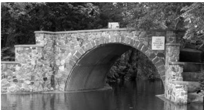
Steel Structural Plate Pipe Arch Installed c. 1940 Inspected in 2012
