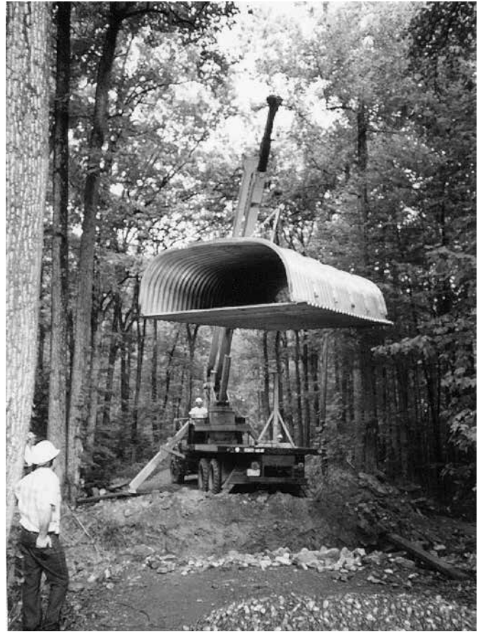
Lifting of Aluminum Box Culvert
