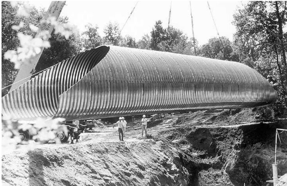
Lifting of Preassembled Aluminum Pipe Arch
