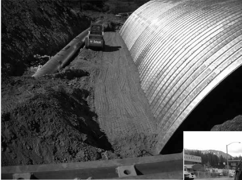
BridgeCor Backfill and Compaction
