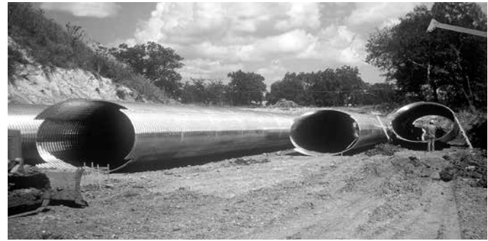
Installation of Aluminum Horizontal Ellipses
