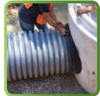
Manhole Boot Connection with Corrugated Pipe Adapter
